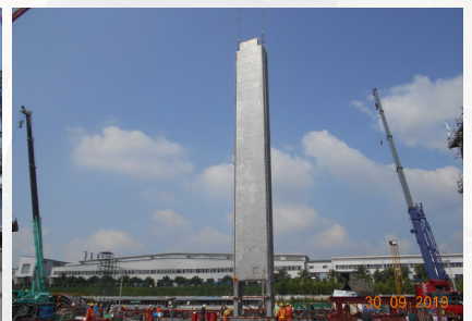
Lifting and install casing wall panel by Crane 400 Ton
